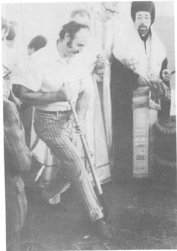
John Eliacostas, then chairman of the building committee turns a spadeful.
